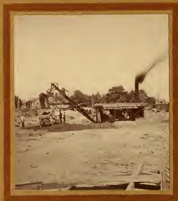
EXCAVATING FOR THE NEW PLATE BUILDING
